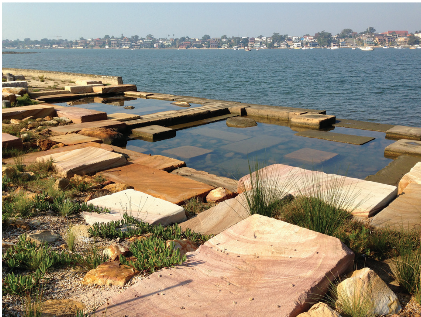
Figure 5. Section of the completed Carss Bush Park seawall including rockpools with integral habitat features and saltmarsh.
