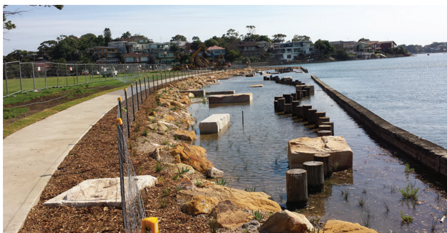
d) Photo Point 2 (PP2 Fig 3) 'after' construction illustrating tidal migration into saltmarsh benches during king tide events.
