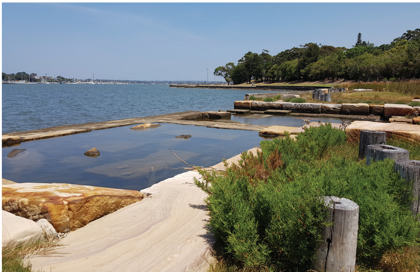
Figure 1. Section of the completed Carss Bush Park seawall including rockpools and saltmarsh.
